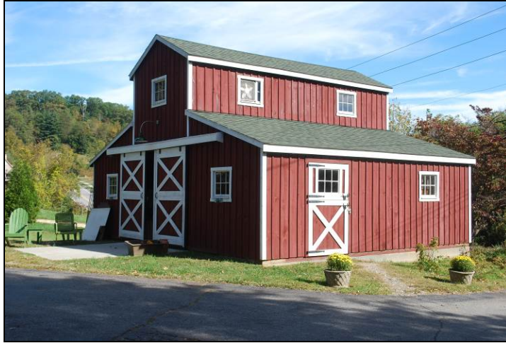
Photograph 85. Prefabricated Storage Shed
