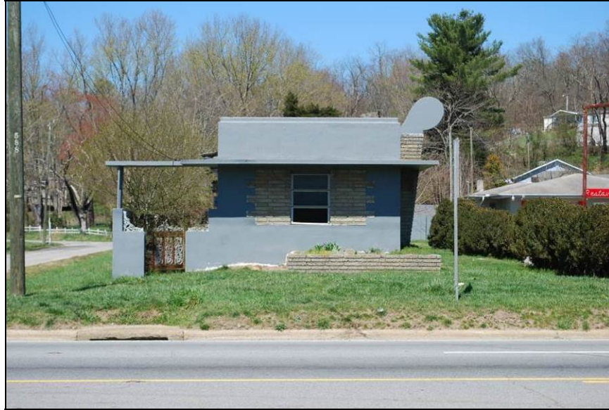
Photograph 12. South Elevation, Building No.2
