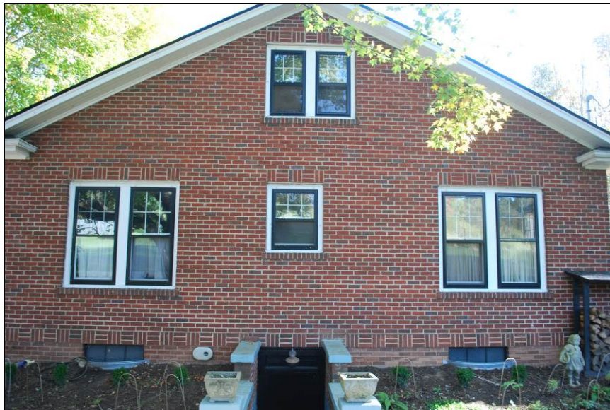
Photograph 80. Roberson Bungalow, rear elevation
