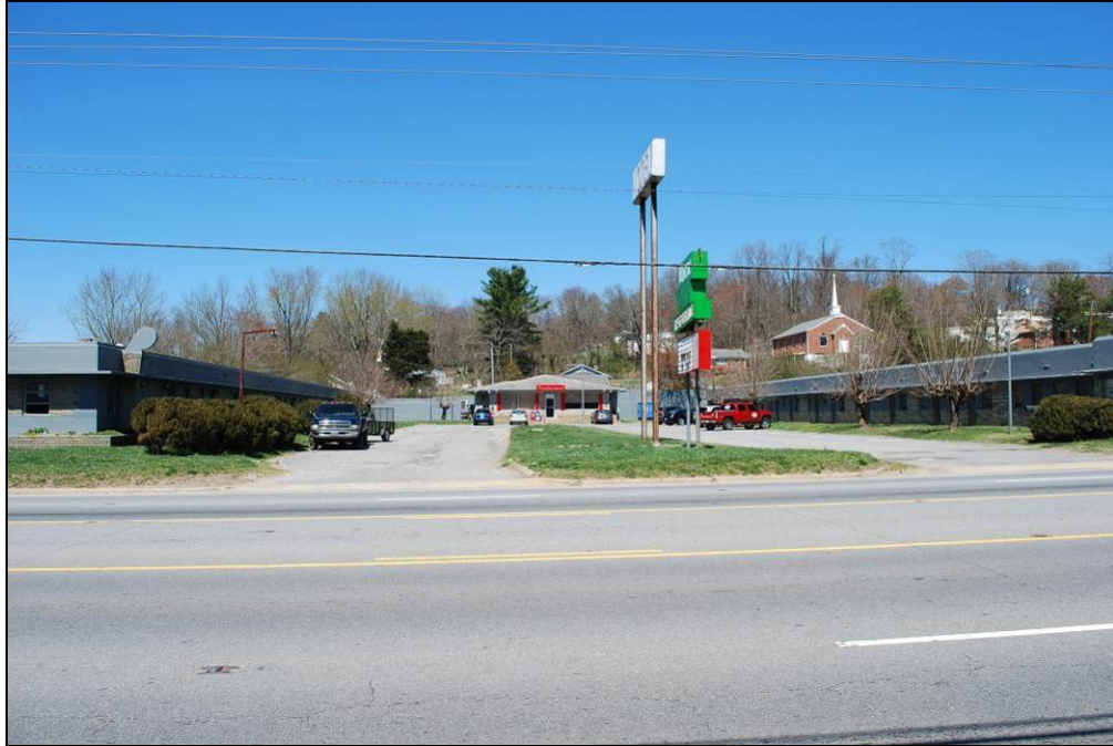
Photograph 1. Overall View of the Miami Motel and Restaurant Property, looking north
