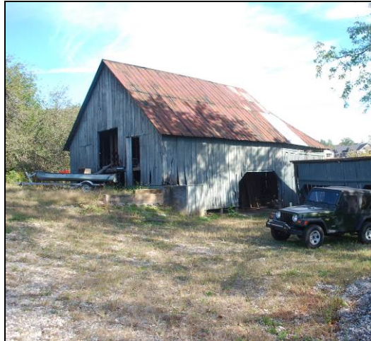
Photograph 92. Frame Barn, southwest oblique
