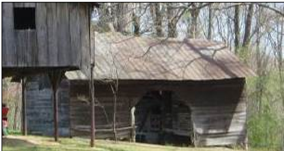
Photograph 67. Double Crib Barn
