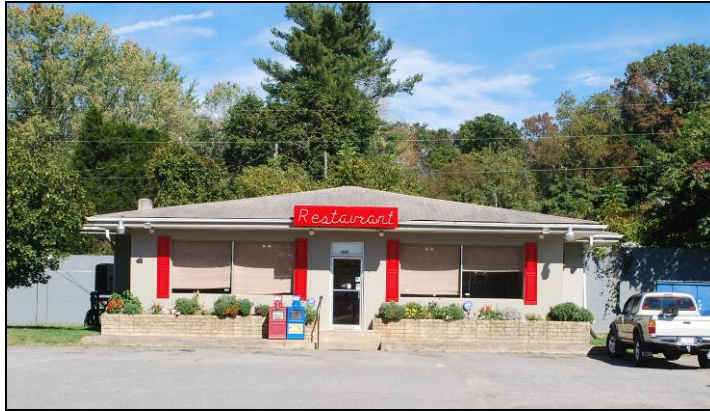
Photograph 15. Miami Restaurant, looking north
