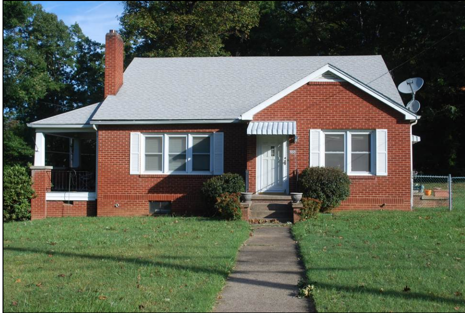
Photograph 49. Liberty Baptist Church Parsonage, Façade
