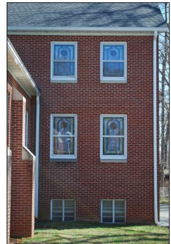
Photograph 30. North Elevation of the West Wing
