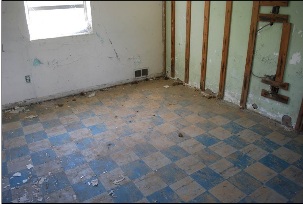
Photograph 8. Interior Room Floor Tiling
