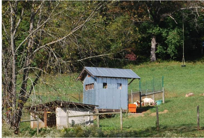
Photograph 89. Shed within Livestock Pen
