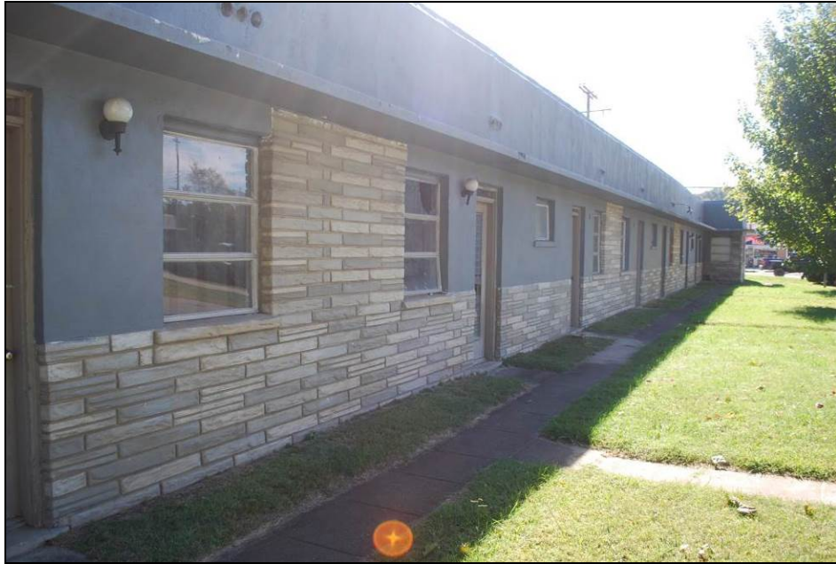
Photograph 4. Façade (west elevation) of Building No. 1, looking southeast
