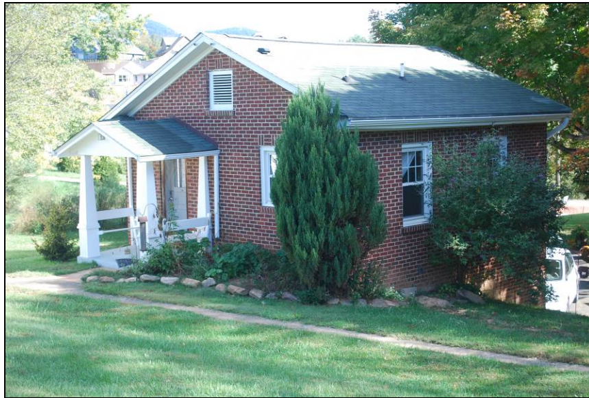
Photograph 83. Garage Apartment, southwest oblique
