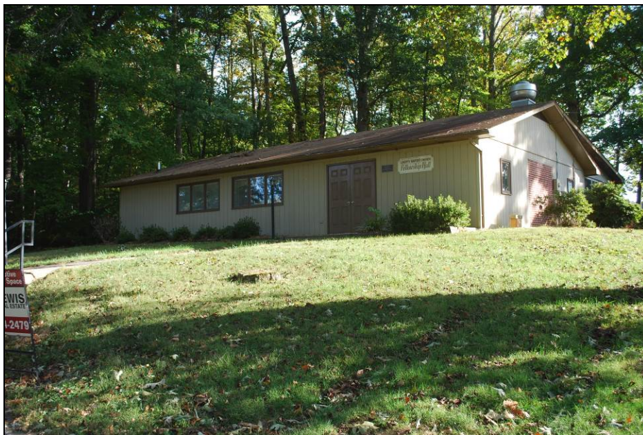
Photograph 54. Southwest Oblique, Fellowship Hall
