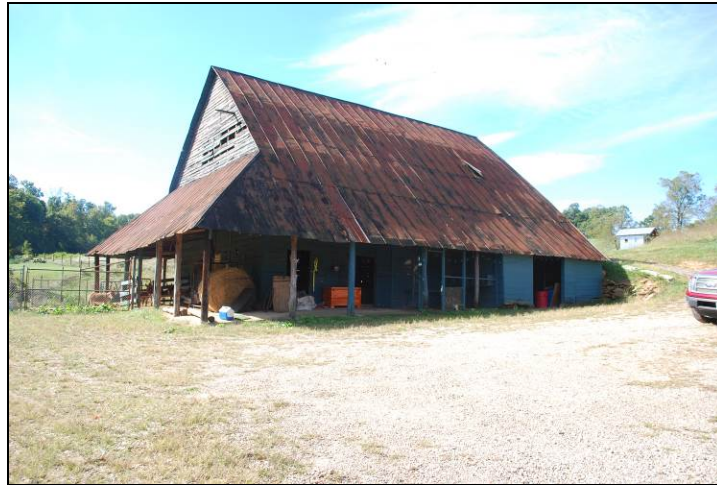
Photograph 90. Dairy Barn, looking southeast
