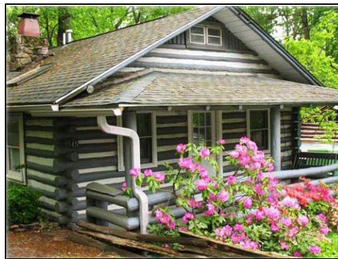
Photograph 68. Homeland Park Cabin
