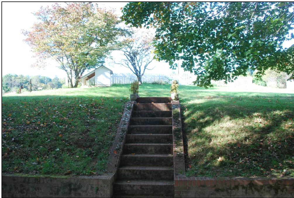
Photograph 71. Westerly View of Brick Retaining Wall and Steps Located at the Rear of the Residence
