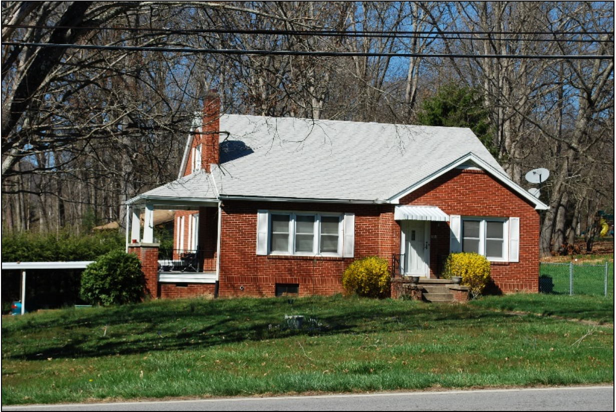
Photograph 48. Liberty Baptist Church Parsonage
