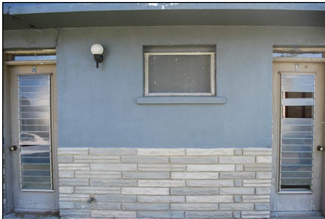
Photograph 5. Glass Jalousie Entry Doors and Textured Glass Bathroom Window
