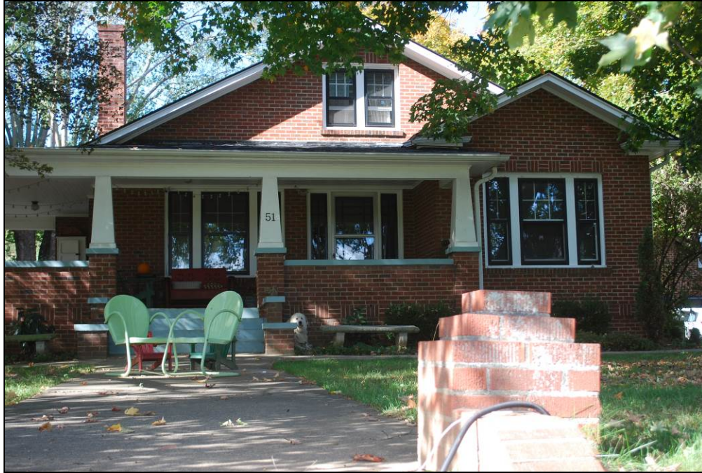
Photograph 77. Roberson Bungalow, façade (east elevation)
