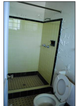
Photograph 7. Bathroom Tiling, Building No. 1
