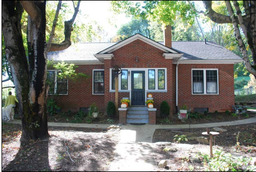
Photograph 81. Roberson Bungalow, north elevation
